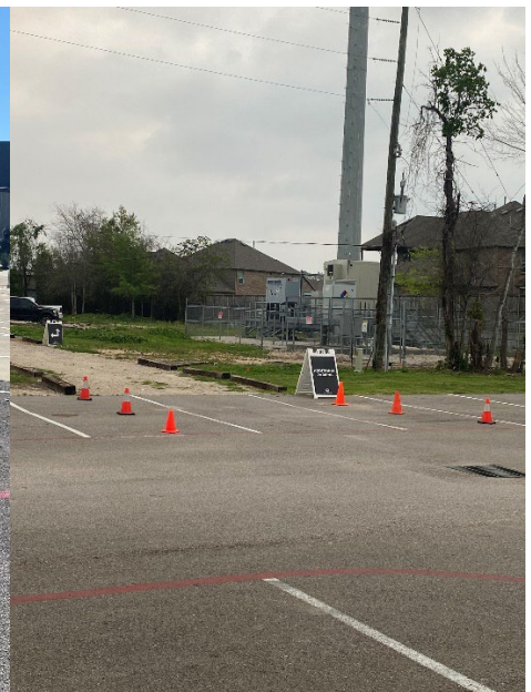
Overflow access w/signs & cones
